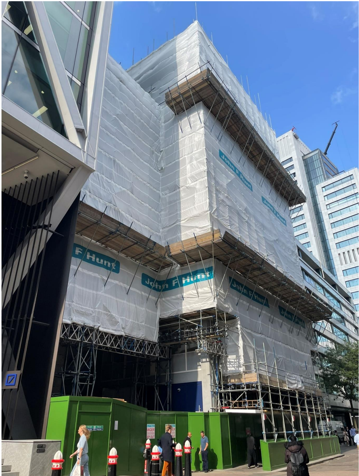
Image 6: East elevation of site from Moorfields – currently under demolition
