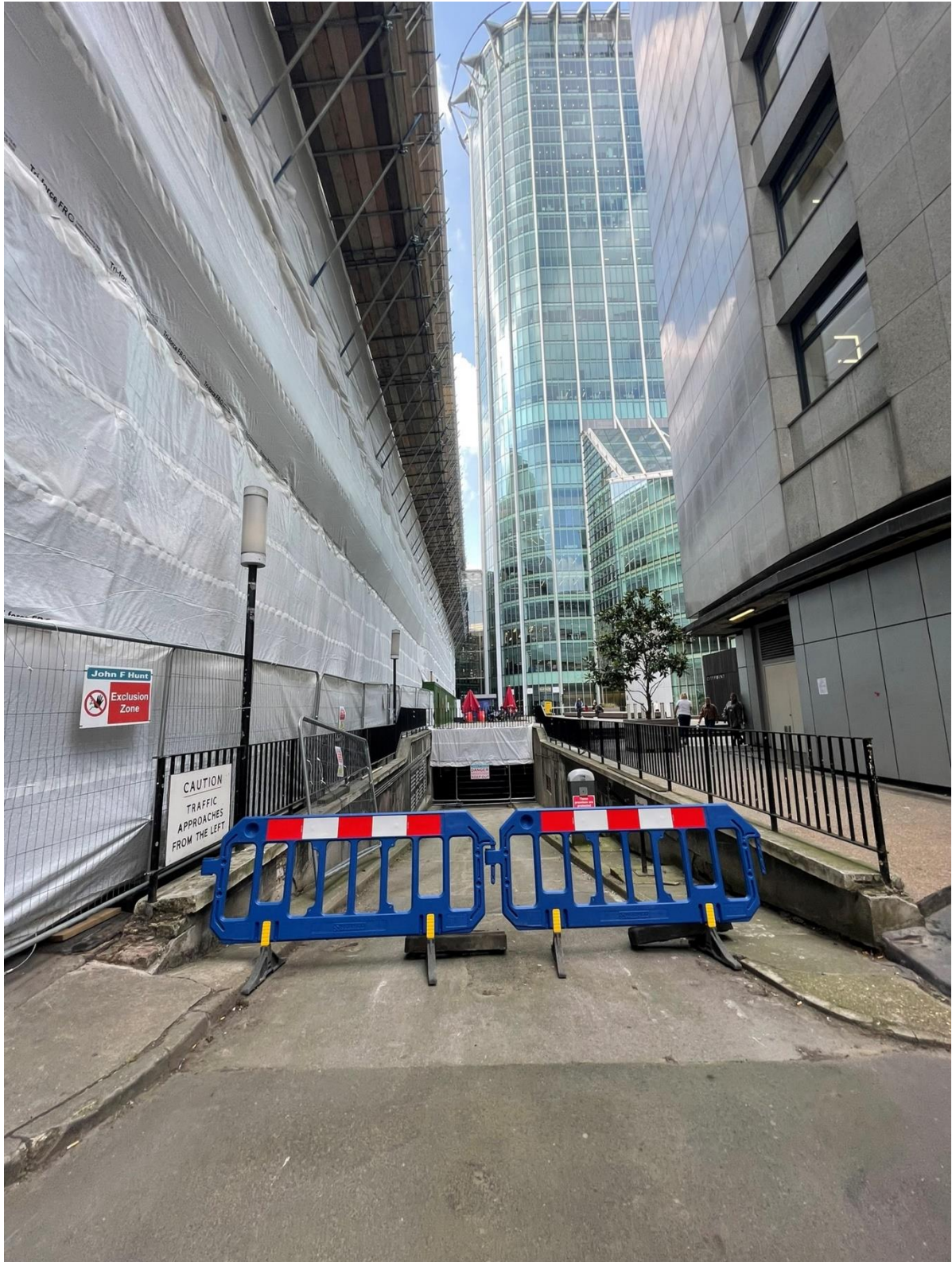
Image 11: Ramp to Plaza to be removed
